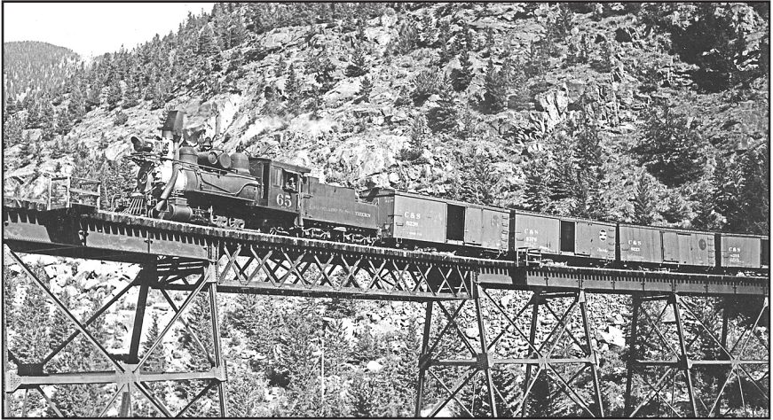
C&S #65 is dropping downgrade on the high bridge at Silver Plume, Colorado, on July 22, 1938. – Henry Griffiths photo from the Carroll Weis Collection.
